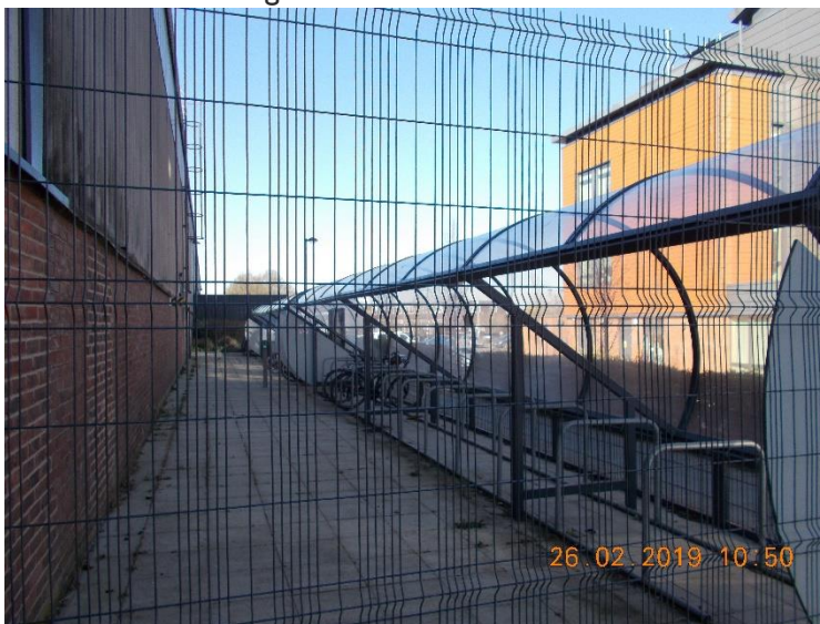
Photo 13.4 Existing West Suffolk House secure sheltered staff cycle parking (2)
