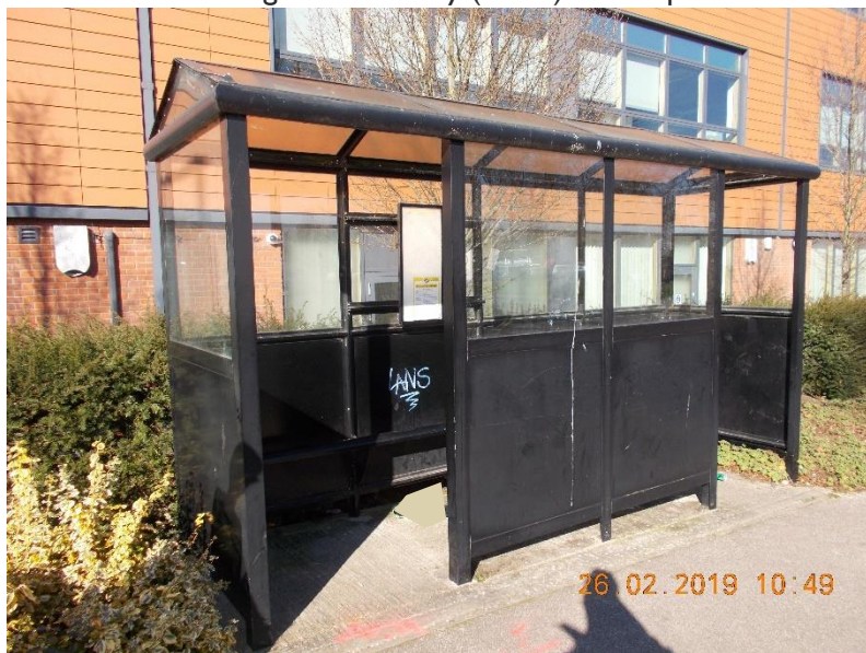
Photo 13.1 Existing Beetons Way (south) bus stop
